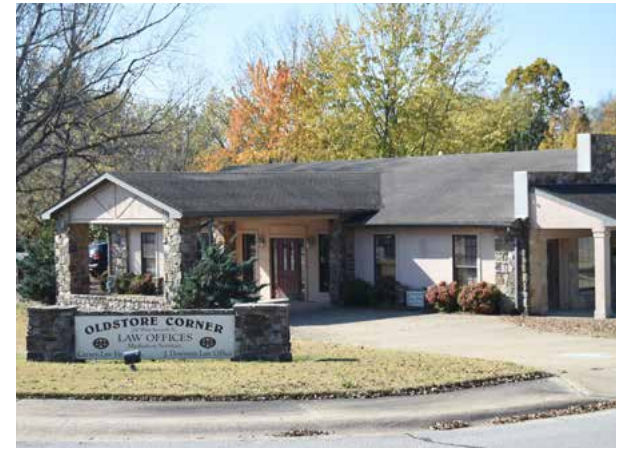
The Carney Law Office, which is closing its doors in December, has been purchased by Baxter County for use by the Sheriff's Office as additional office space. SCOTT LILES/THE BAXTER BULLETIN
